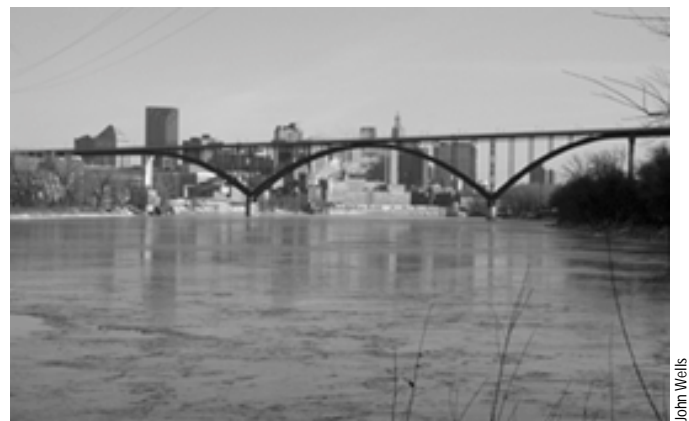
St. Paul's High Bridge
