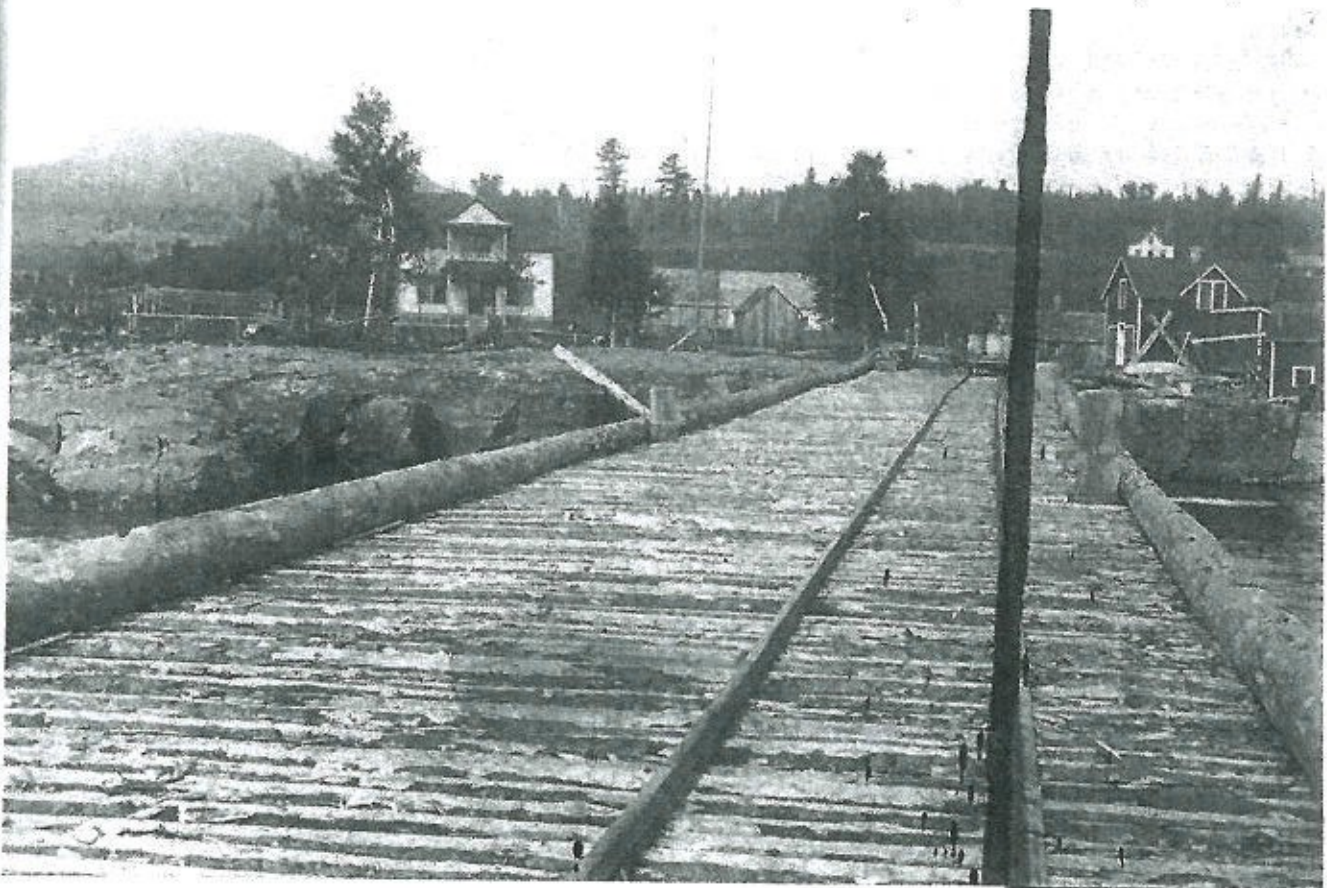
This damaged photo of Tofte was taken in 1908-9. The central feature is the log and cribbed dock built eight or nine years earlier; note the rails and cart in the distance with a load of barrels. Carlton Peak is in the background. The conspicuous white building is Hans Engelsen's Homestead Hotel; the structure on the right housed his store and Post Office. That white home in the distance belonged to the Helge Tofte family. By 1915 this dock had become inadequate; it was replaced by a concrete structure in that year. From the photo collection of Ted Tofte.
