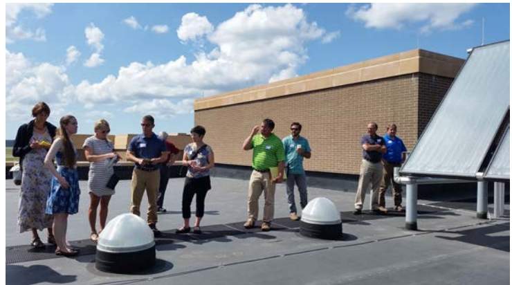
2016 Minnesota GreenCorps energy conservation member leads a rooftop tour showing off installed Solatubes and solar thermal panels that add to Camp Ripley's resiliency while reducing greenhouse gas emissions. Source: MN Pollution Control Agency
