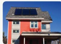
The first Twin Cities Habitat for Humanity Net Zero home in north Minneapolis is built to the highest levels of energy efficiency, insulated at least three times as much as a regular house and sealed extremely well to keep drafts out.
