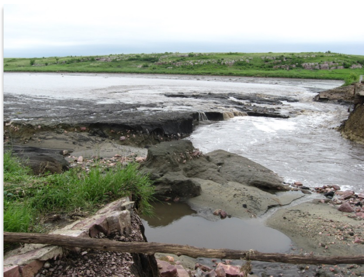
FIGURE 12. DAM AT BLUE MOUNDS STATE PARK, JUNE 2014
