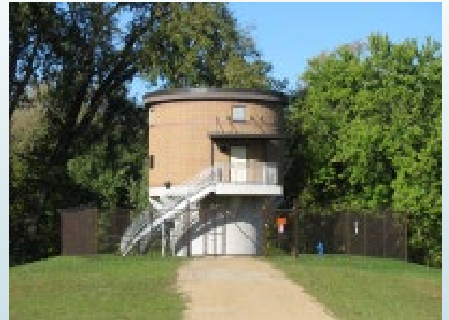
Shallow collector well – 75% of city's water supply comes from 2 collector wells influenced by Minnesota and Blue Earth Rivers
