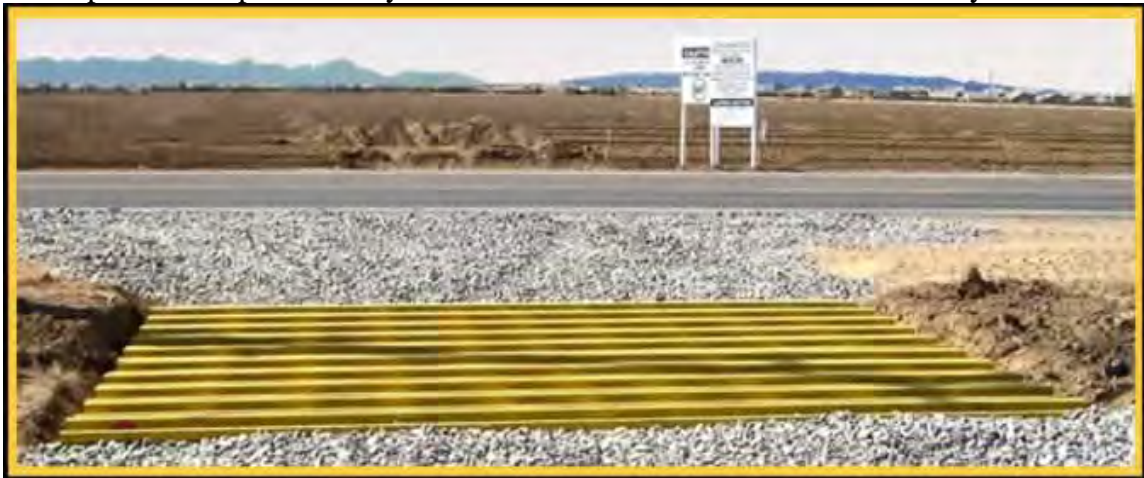
Figure 5. Grizzly pad used with gravel pad.
