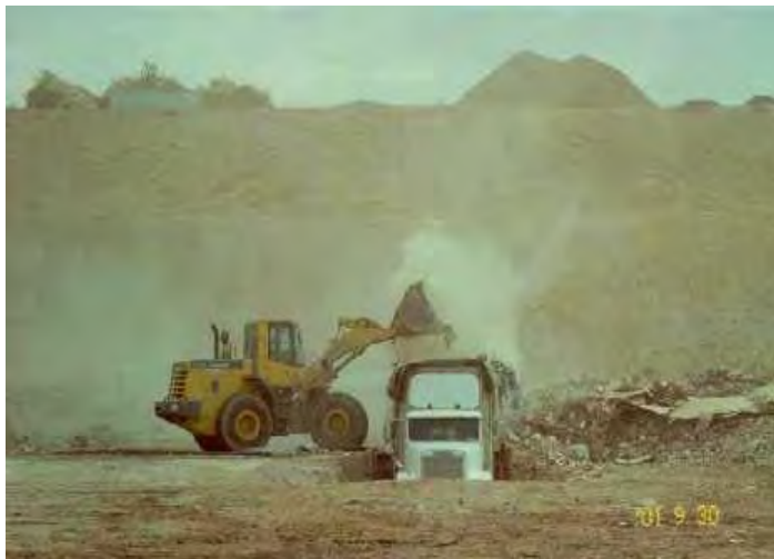
Figure 11. Loading operation without dust control measures
