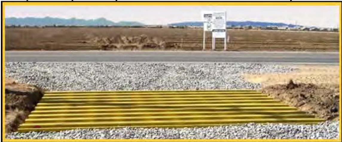
Figure 5. Grizzly pad used with gravel pad.
